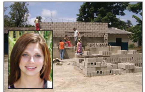
Amphitheater construction. Inset: Amy Polomsky.
