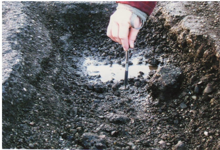
Photograph of a portion of the actual pothole at the accident scene taken by the Ohio State Highway Patrol.
